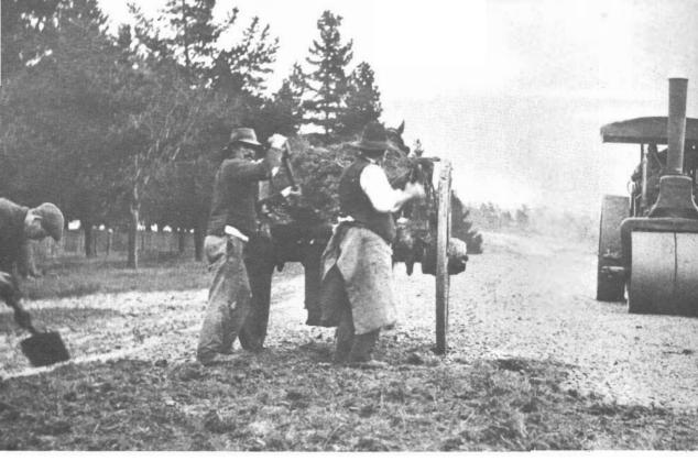
Dandenong Road in 1913. A form of road construction using metal, soil, weeds, and grass to provide a surface.
